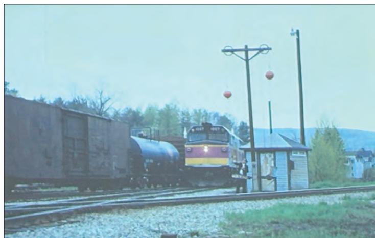
The lowering of the ball signal at Whitefield.
